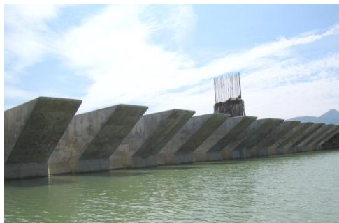
Figure 4: Van Phong under construction
