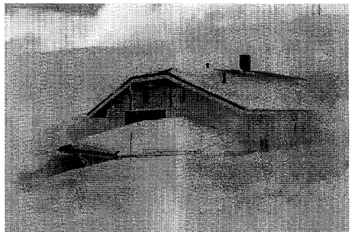
Figure 4. Building covered by drift snow in the south-west end of residential area IV in Fuglenesdalen, April of 1997. This section is open for snow drift from south-west.
