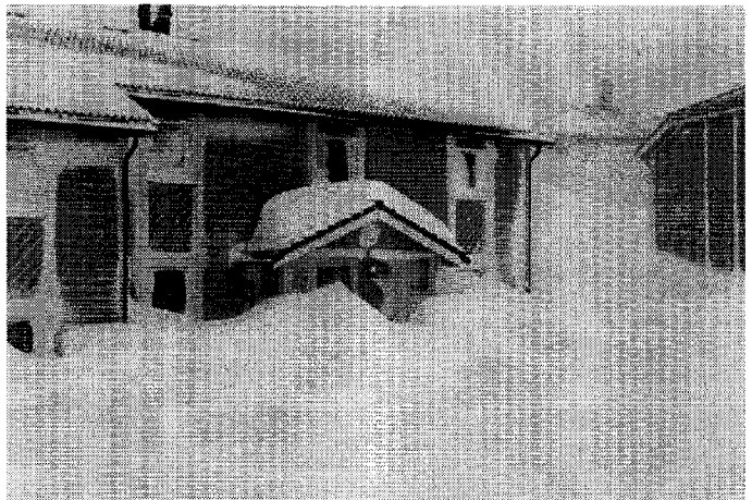
Figure 2. Snow drift in the south-west section of residential area IV in Fuglenesdalen during a snowstorm in April 1997.
