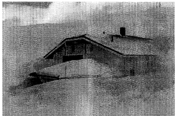
Figure 4. Building covered by drift snow in the south-west end of residential area IV in Fuglenesdalen, April of 1997. This section is open for snow drift from south-west.
