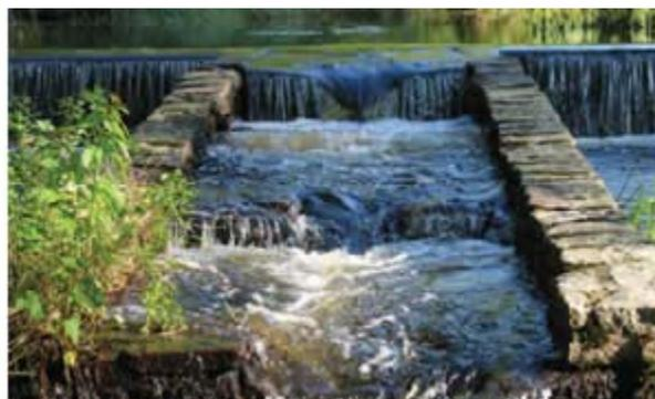
**Fig 1:** The deteriorated fish ladder: The image on left is the calculated flow configuration, while an actual photograph at right shows damaged lower weirs.
