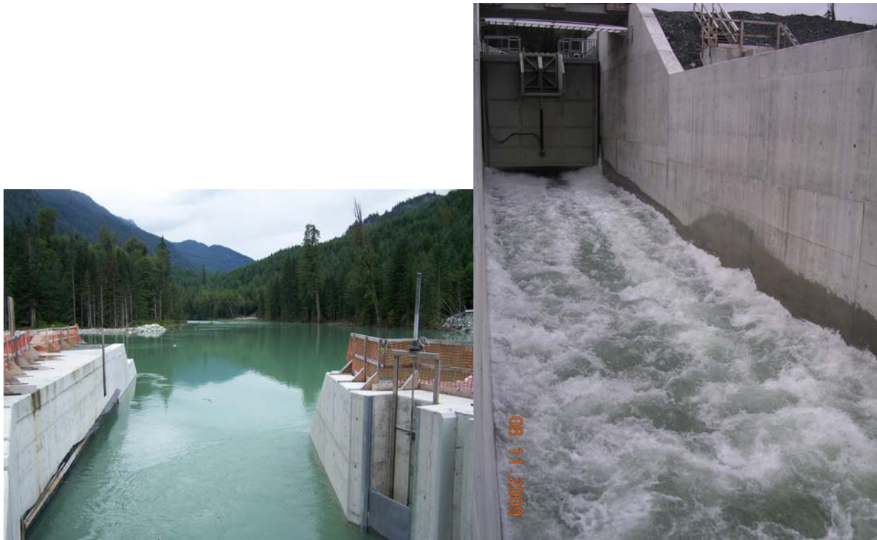
Figure 9: Ashlu Creek Sluiceway in operation ( 50 \text{ m}^3/\text{s} ) Entrance of the structure (left) and gate opening (right)
