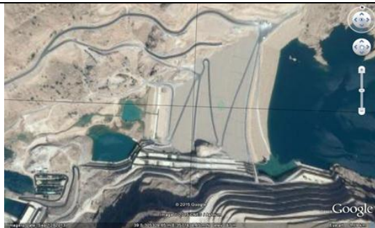
Figure 1. Upper Gotvand Dam.
